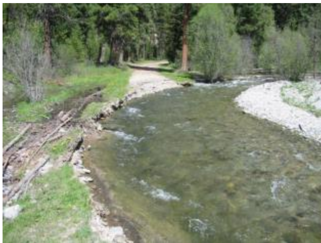
Figure 2.2F. Washed out portion of the county road below a newly installed bridge, following flood events in spring of 2009.
