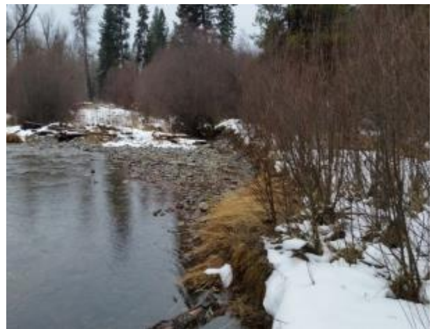
Figure 2.2G. Washed out reach of the county road (opposite direction as Figure 6.1E) that has been revegetated.
