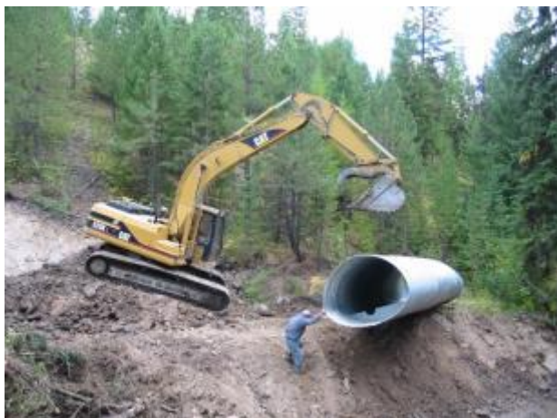
Figure 2.2H. Baffled fish passage culvert being lowered into place in a tributary to Big Rock Creek in 2003. Photo credit: WY.
