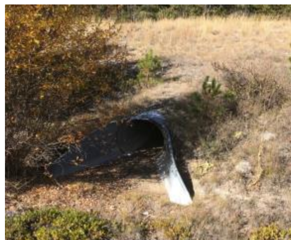
Figure 2.7J. Culvert that directs highway runoff and sediment load towards McGregor Creek.
