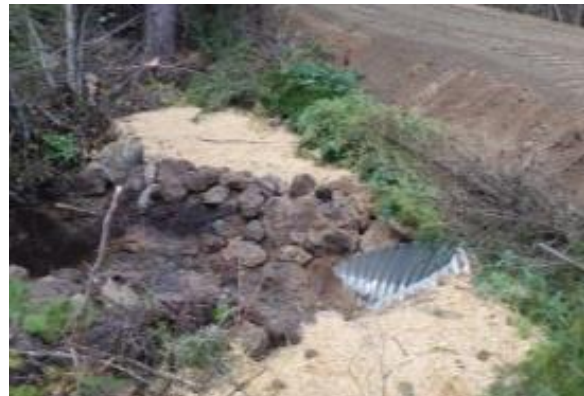
Figure 2.5G. Stream crossing culvert upgraded by WY for fish passage on tributary to Mudd Creek in 2016.
