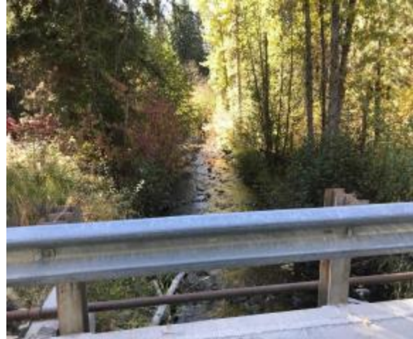
Figure 2.7F. Looking downstream on McGregor Creek after it passes under bridge on Thompson River Road.
