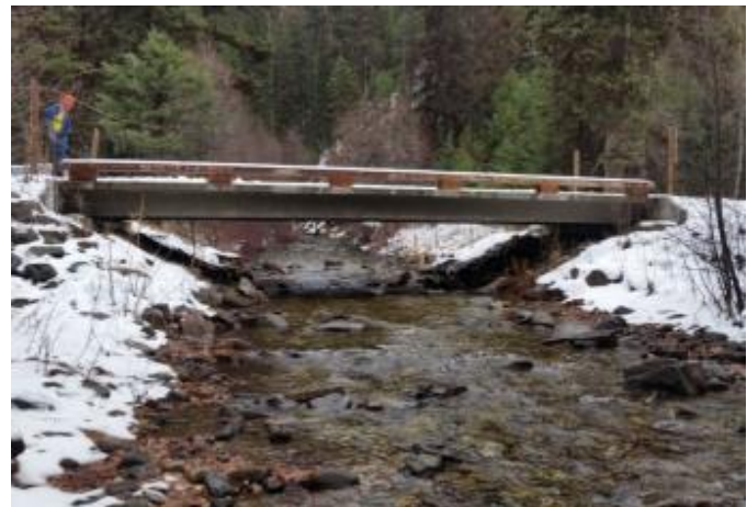
Figure 2.2I. Bridge over Big Rock Creek on the county road installed in 2009 (or 2010).
