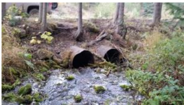
Figure 6.8B. Big Hole Creek culverts (Big Hole Creek confluence with Thompson River) prior to upgrade (2016 photo). Photo credit: Ryan Kreiner.
