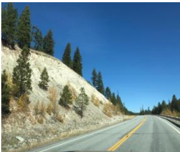
Figure 2.7I. Current cutslopes along US Highway 2 that is eroding and a potential source of sediment to McGregor Creek.
