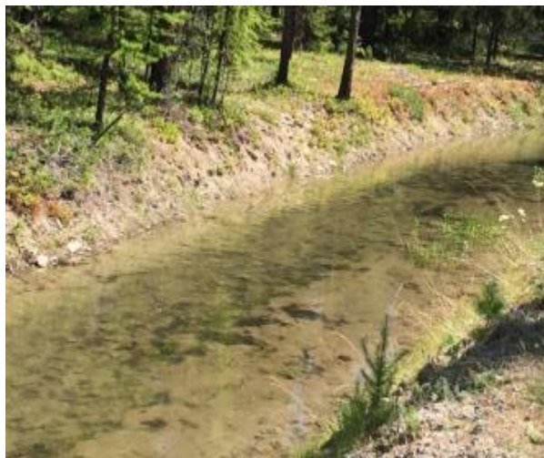
Figure 2.5B. Alder Creek ditch directing water from Little Thompson River to the Flathead Reservation.
