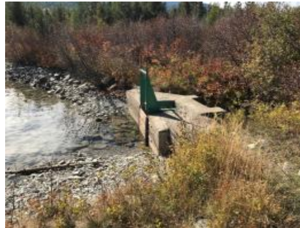
Figure 2.7B. Irrigation control dam/headgate at outlet of McGregor Lake.
