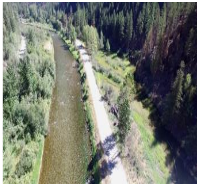
Figure 2.8A. The Thompson River is closely paralleled by CR 56 and FR 9991. Photo Credit: Paul Parson (TU).
