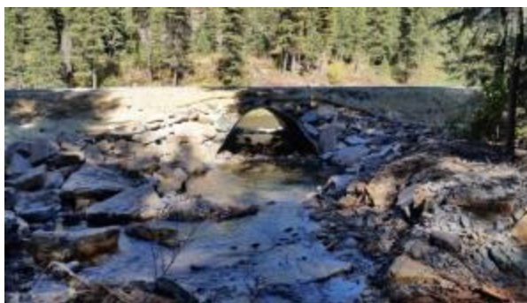
Figure 6.8C. New crossing on ACM road of Big Hole Creek. Installed by USFS-LNF in 2017.
